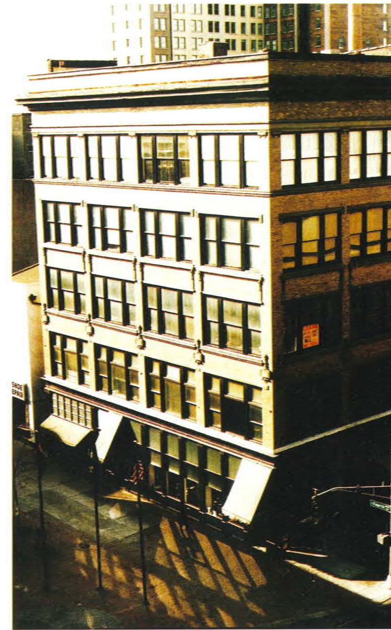
The Norton Building at 200 Fourth Avenue, Louisville, Kentucky.
